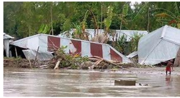
Fig. 1b: Collapsed Building due to a typical Effect of Floods in Community
